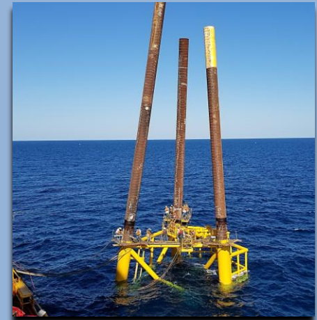
Offshore Platform Installation
